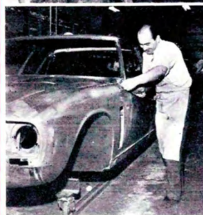
A story in pictures: the completed chassis passes to the body pressing jig. The doors and boot lid are fitted by hand before the completed bodyshell is finished and cleaned for painting. The bottom picture shows the bodyshell rising from the first paint dip.
